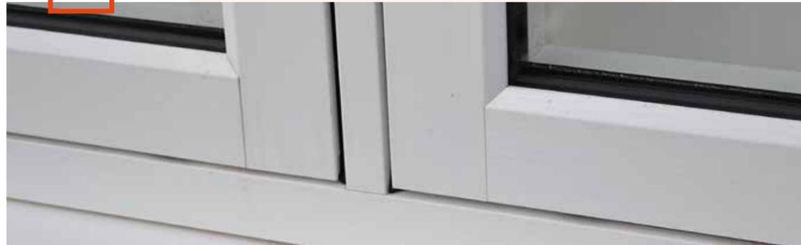
A mitre weld will fuse the joints together diagonally for a contemporary appearance, or choose the Graf weld for a seamless diagonal weld. The Timberweld® process welds the profiles with a mechanical look to both sides, or MechWeld/ External Timber Look (ETL) gives a diagonal weld to the internal, with a mechanical look to the external. Of course, there's also the traditional mechanical joint which is not welded, but made in a traditional mechanical jointed method, often used in timber joinery.
